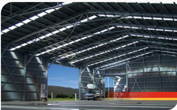
Large Span Structure
